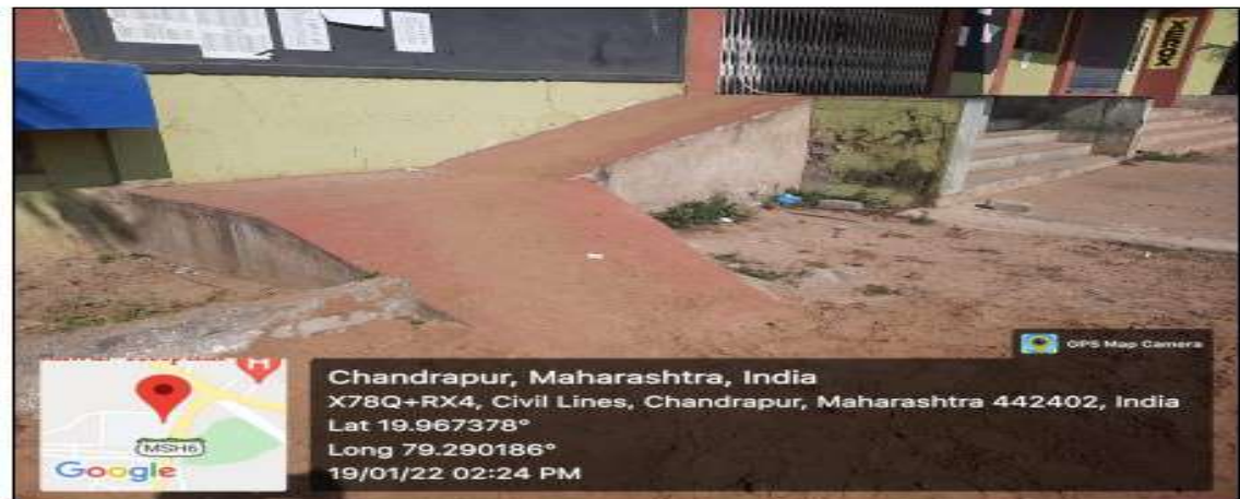
Ramps to facilitate Differently Abled
